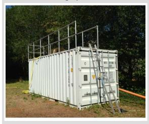
The focus of the comparison was on the reduction of secondary sludge. The scenario was a mobile treatment plant in container design that was operated in parallel with a capacity 2 treatment plant. Split into two project phases, the activated sludge process and the biofilm process were observed separately from one another. During the biofilm process, the carrier material of EMW<sup>®</sup>, Poret<sup>®</sup> aqua, was used.
