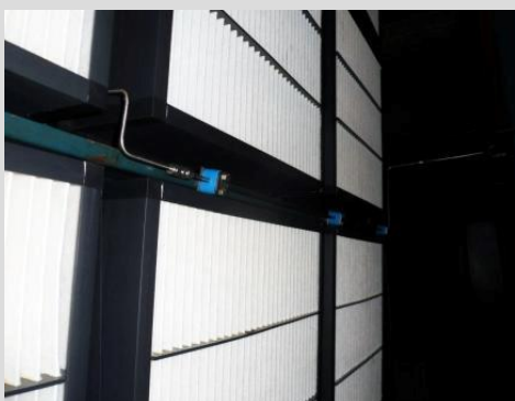
The picture above shows an installation of the Z-Line GT in a filter house at UK. As easily applicable at the existing frame system, EMW® has installed a version with a header frame. Presently the pre-filter cell is close-coupled in front of EMW®'s Minipleat GT Compact Cassette F8 (MPK48 - 20 GT).
